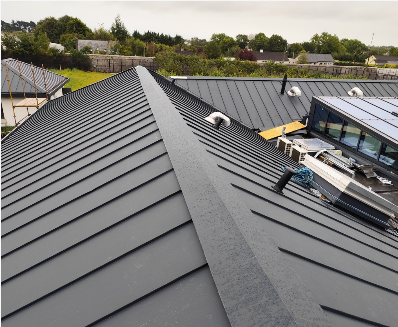
COMPLETED STANDING SEAM ROOF
