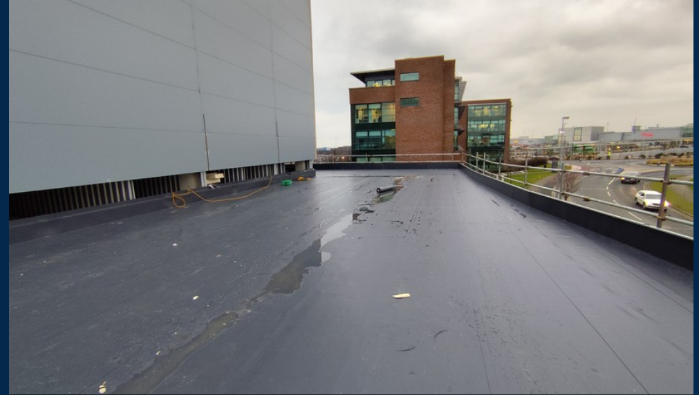
MEMBRANE COMPLETION STAGE
